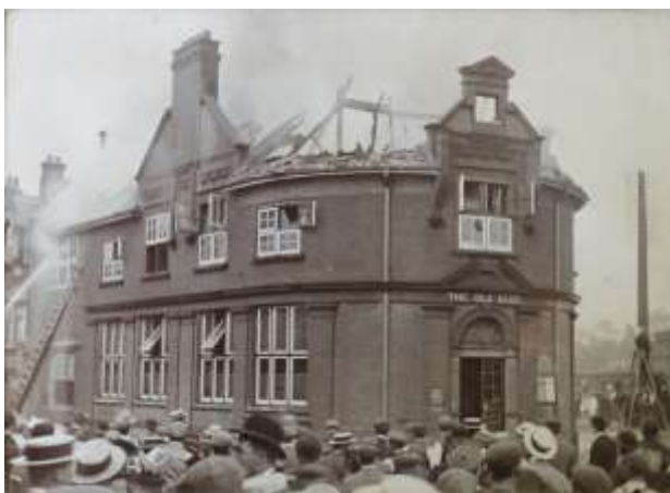
Figure 16. Fire at Council Offices
