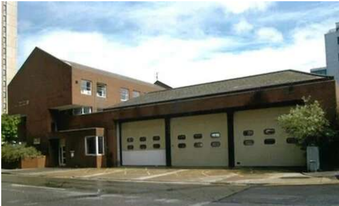
Figure 38. New Church Street station, built 1981
