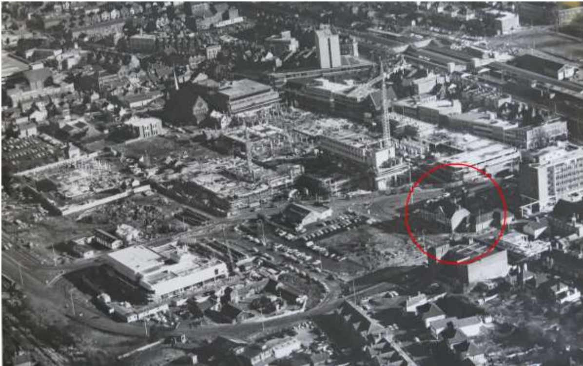
Figure 35. Church Street station surrounded by desolation c.1973
